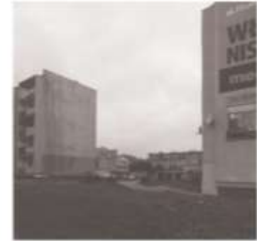
unfinished block structures
