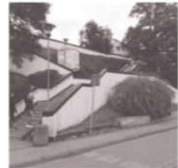
connecting tthe upper terrace
